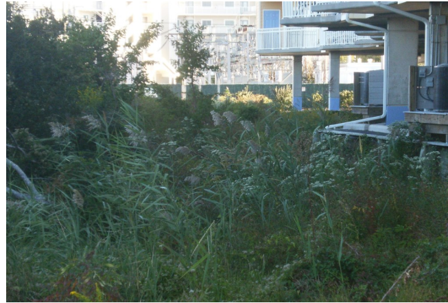
Stormwater treatment facility Critical Area buffer, Ocean City, Maryland
