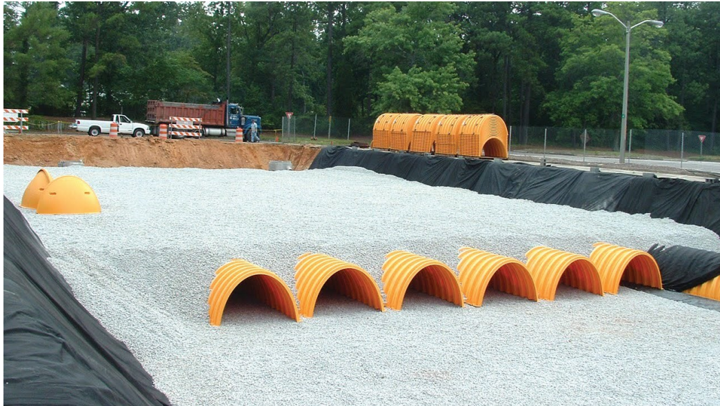
Advanced Drainage Systems Inc.—StormTech Chamber System Installation
