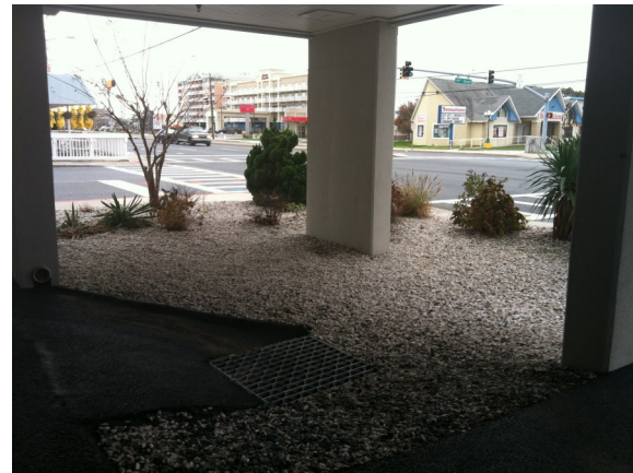
Parking lot runoff to stormwater treatment area Ocean City, Maryland
