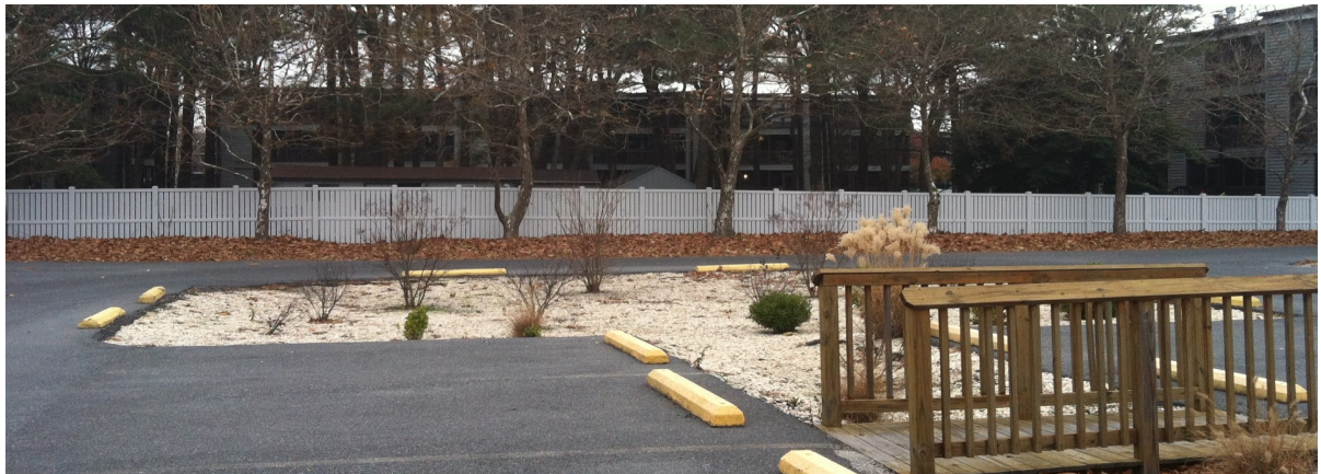
Stormwater treatment facility Ocean City, Maryland
