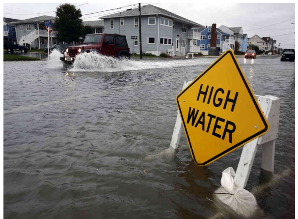
Tidal water over roadway during Hurricane Sandy South Ocean City, Maryland
