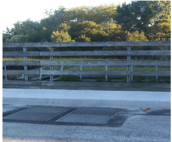
Catch basin within Critical Area buffer Ocean City, Maryland
