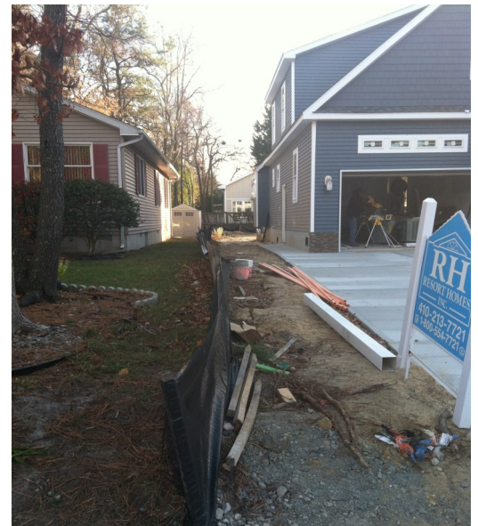
Single-family home construction with Erosion and Sediment Control, Ocean City, Maryland
